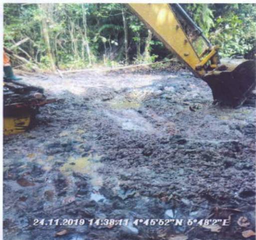
Fig A: picture taken before excavation.
