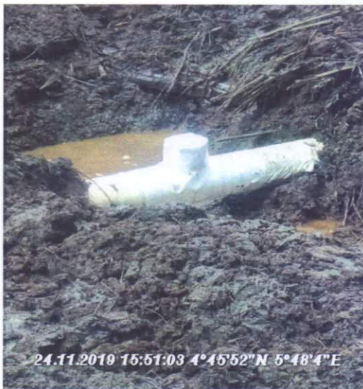
Fig C: picture taken after wrapped.
